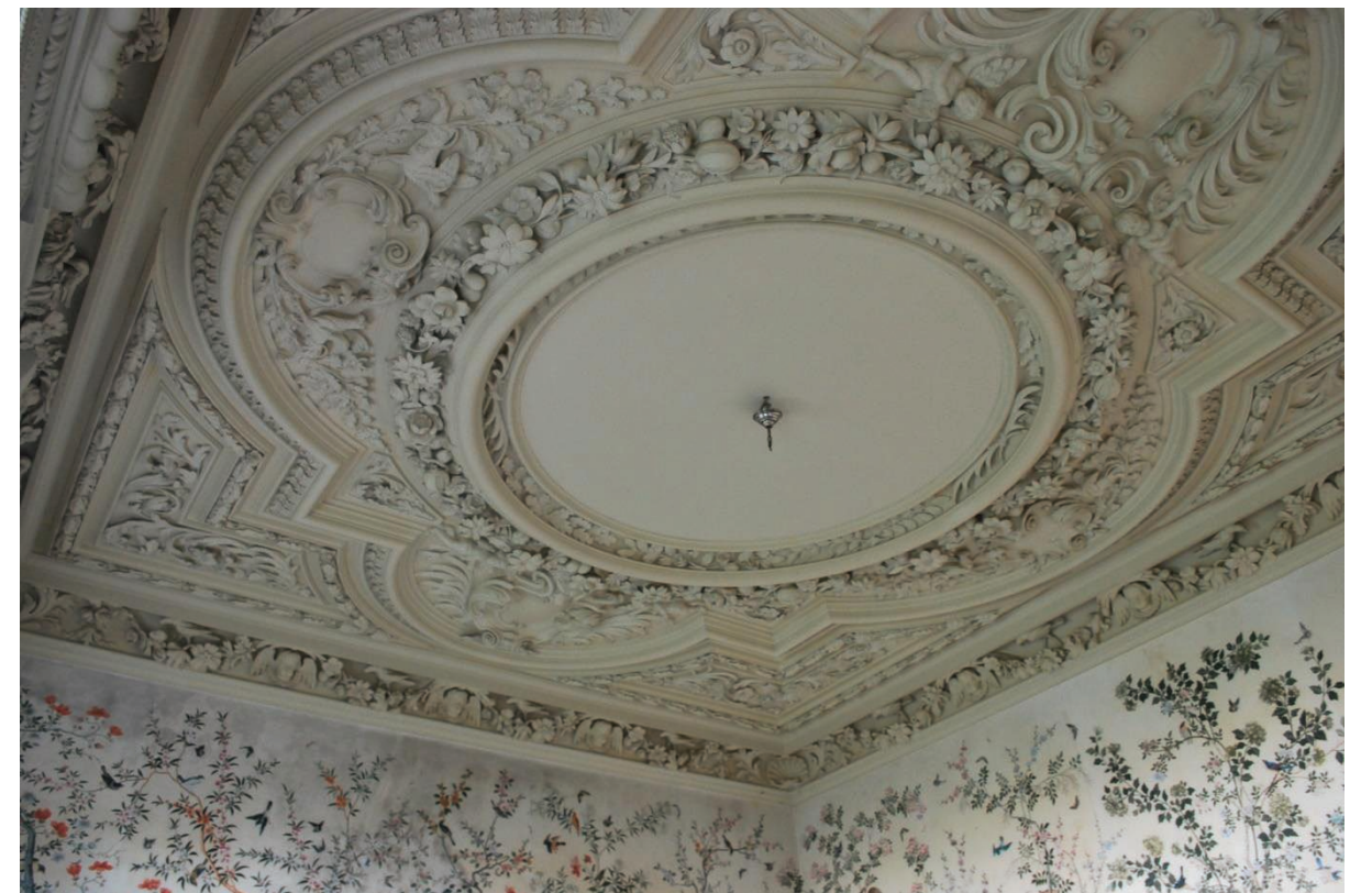
Fig. 5.19. The c. 1689 plaster ceiling design, re-cast c. 1926, in the north-east corner first-floor room.
