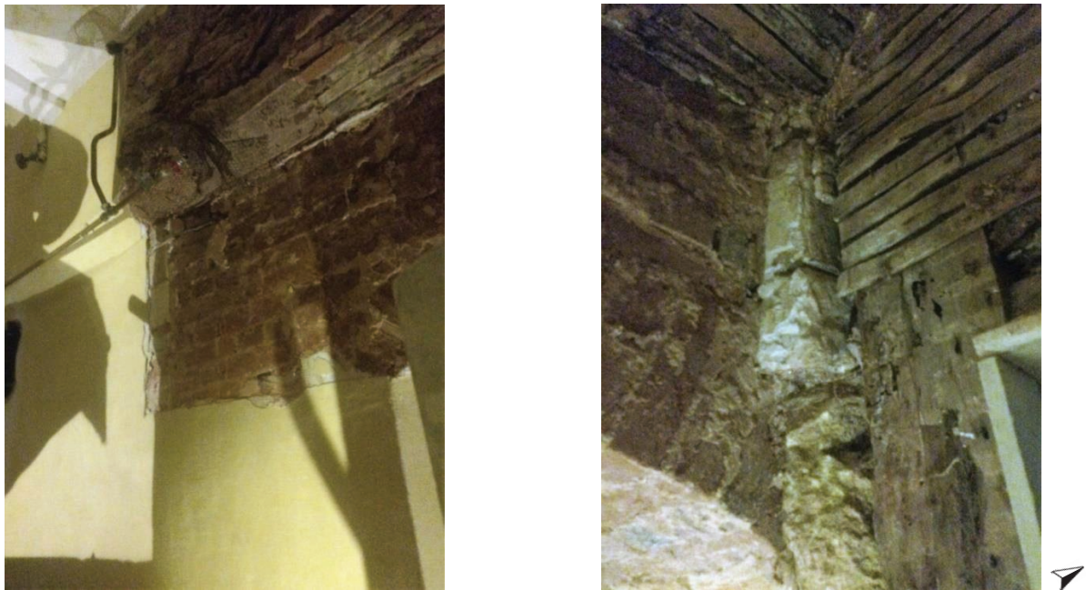
Figs. 3.12 and 3.13. The removed c. 1590 first-floor window left and right upper corners, from within its c. 1590 staircase gable.
