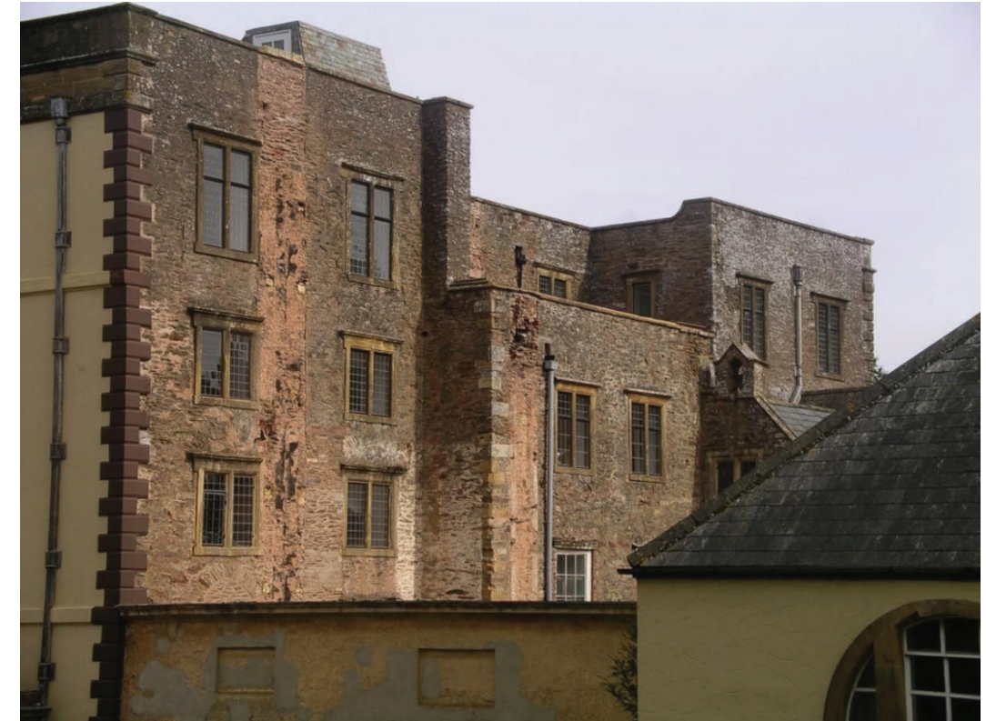
Fig. 5.6. South elevation: showing two vertical scars of removed chimneys from the now demolished Servant's Hall and a repurposed butler's pantry.
