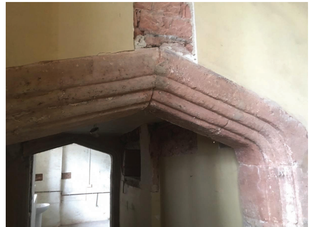
Fig. 5.15. Two early door surrounds in the Hall, with similar cross-section profiles as the cellar door.
