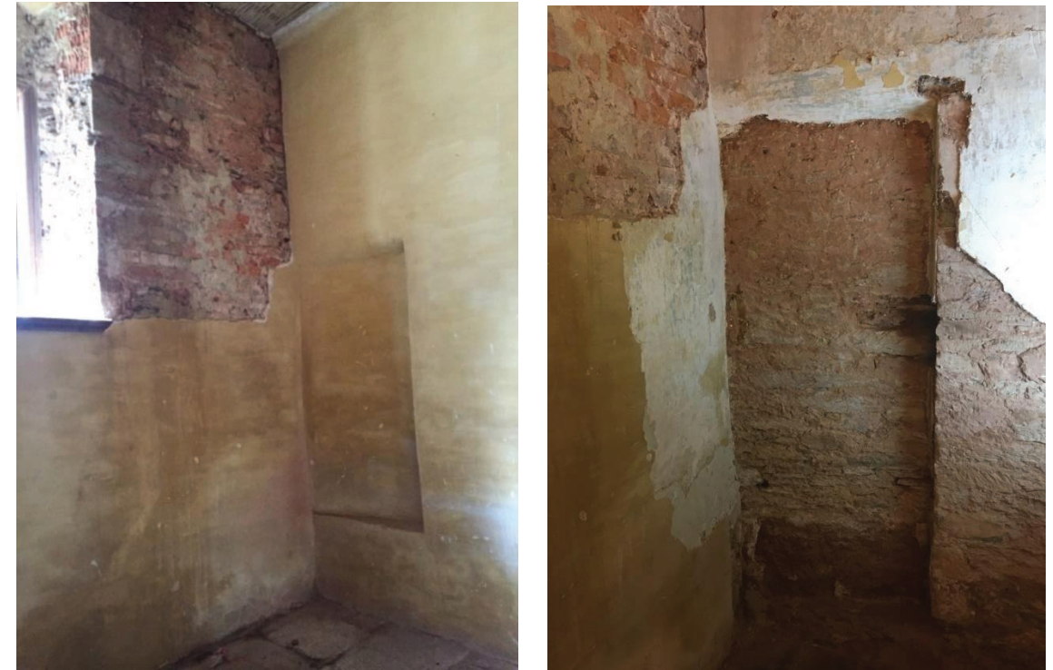
Figs. 3.20 and 3.21. In-filled opening in the north wall of the north gable, with and without modern plaster. The half-door and angle of the opening suggests a spiral staircase but without invasive examination the nature of the area remains unknown. The area to the west wall, right of the window, has been in-filled with redbrick suggesting a larger opening at this corner.
