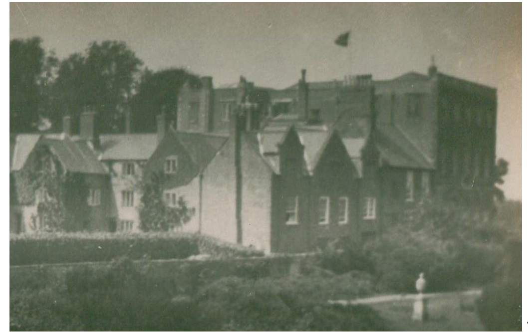
Fig. 2.26. Photograph c. 1908, the east range still with sash windows while mullioned windows had already replaced at least two sash windows in the south range.
