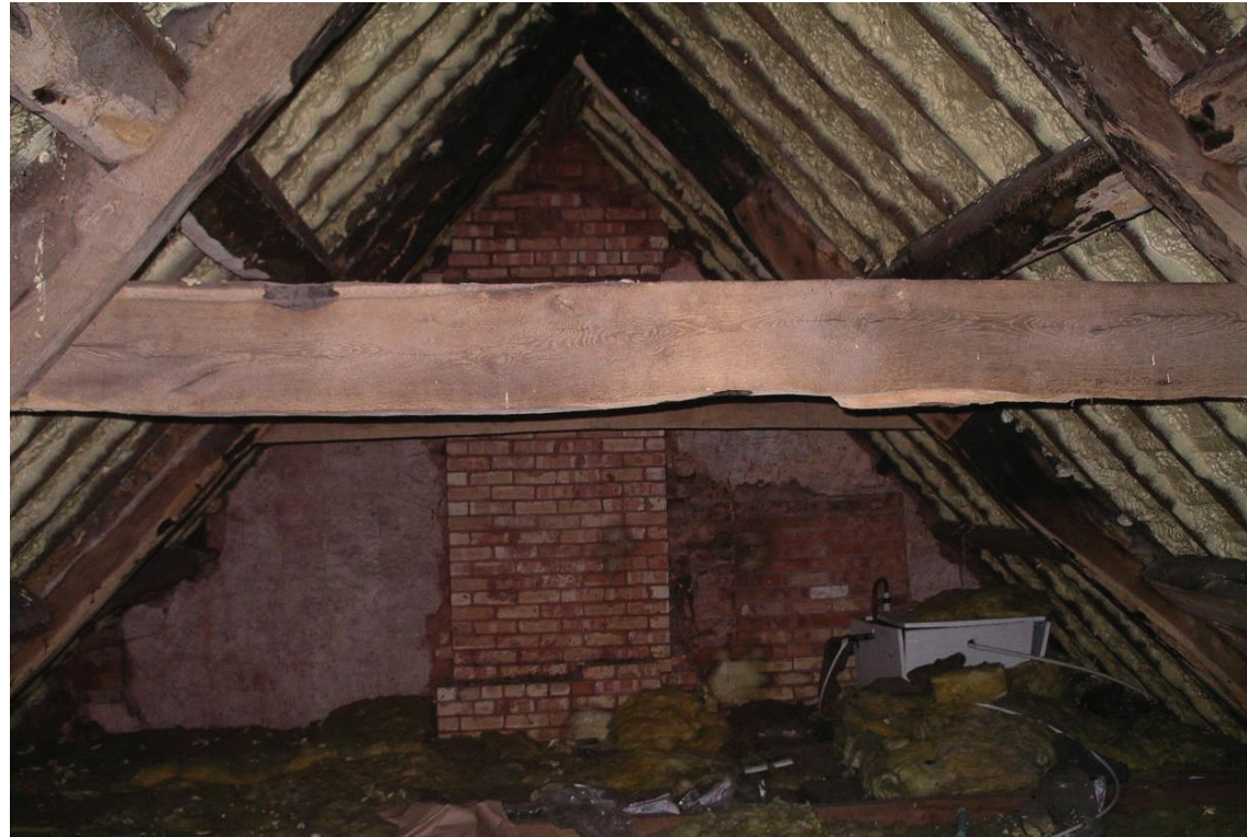
Fig. 4.5. South-west wing attic looking north to a later red brick wall with an in-filled door to the left.
