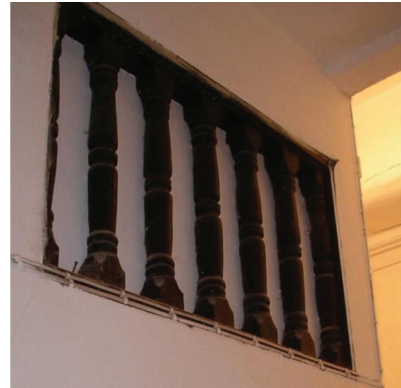
Fig. 3.1. One of four turned-oak baluster sections in situ at the south of the western extension.
