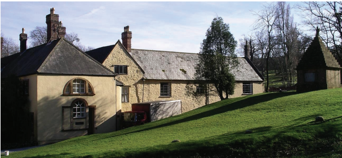
Fig. 4.9. West elevation with natural landscape contour which once abutted the building's wall necessitating access at this elevation only from the first floor.
