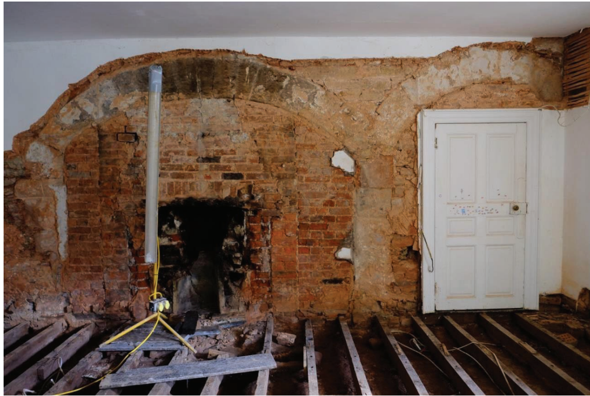
Fig. 3.2 The broad arch of the newly exposed sixteenth-century service fireplace with bread oven to its left and door arch to the right, leading to the service passage behind this fireplace and to the Buttery in the, now attached, two-bay gabled section to the east.
