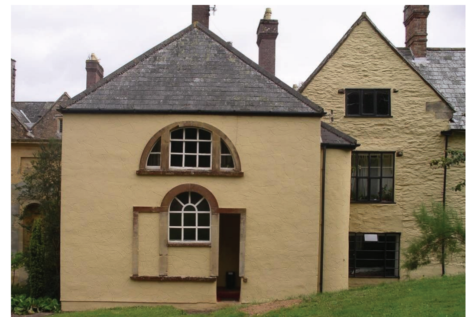
Fig. 4.1. Single-bay, two-storey below an attic extension of rough stone with twentieth-century Crittal windows, a 1754 Palladian addition overlaps from its north.
