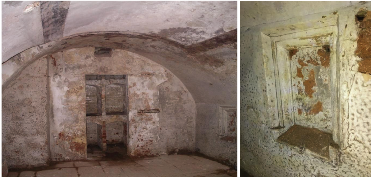
Fig. 5.9. Cellar, southern chamber, west wall, with a hatch surround to the north and a blocked opening in the ceiling to the south.
