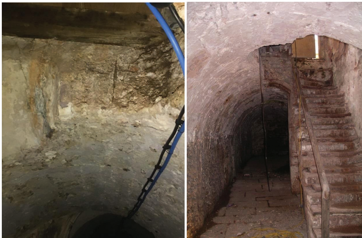
Figs. 5.12, 5.13 and 5.14. The cellar door apex and views of the intersecting tunnel displaying the full thickness of its ceiling structure.
