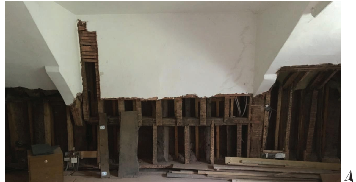
Fig. 2.29 Unusual construction between the north to south aligned single-bay section and the subsequently re-aligned east to west two-bay section. See Plan 3.7 for location key.
