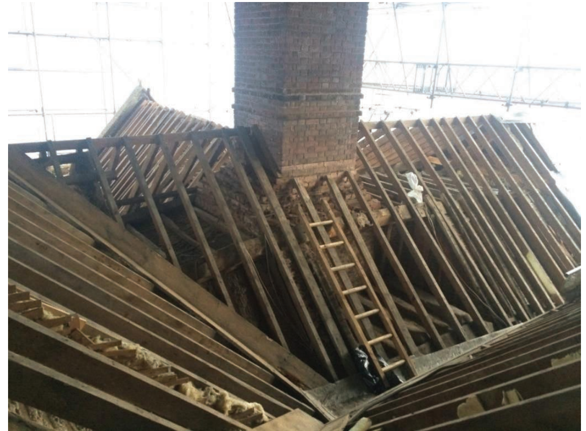
Fig. 2.31. The c. 1590 chimneystack at the east of that later range, see plan 2.6. The purlins supporting the ceiling of the new east facing gable on the earlier east range have sagged considerably from supporting the weight of the east range's older north to south roof alignment.
