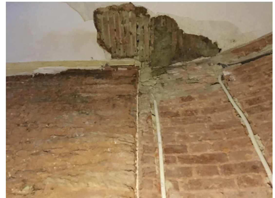
Fig. 3.27 The quoins, returning plaster and returning running rib cornice of the central gable section, with a later red brick partition added to the right.
