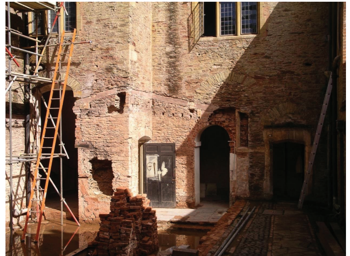
Fig. 3.11. North and central gable sections c. 2005, with the eighteenth-century openings exposed during the demolition of the Servant's Hall. There is a 1771 door opening through the south wall of the north gable. A lower-right horizontal section of the original central gable window still existed, touching the door's left jamb; the upright mullion was reused in its position.
