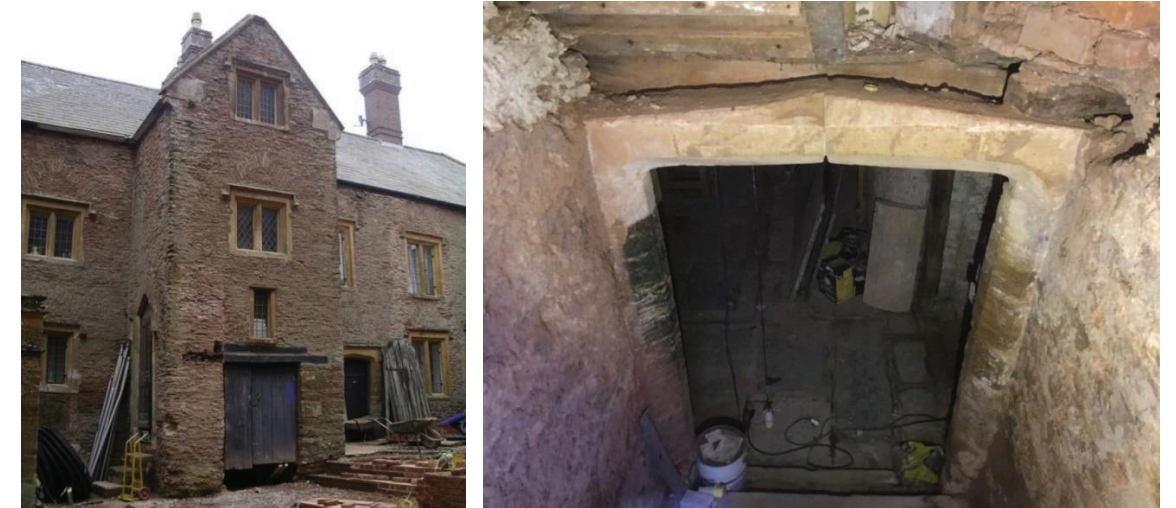
Fig. 3.3. South range, north elevation, c. 2008: stair tower with north cellar entrance and east entrance to floors above, to its west a four-centred arch door.
