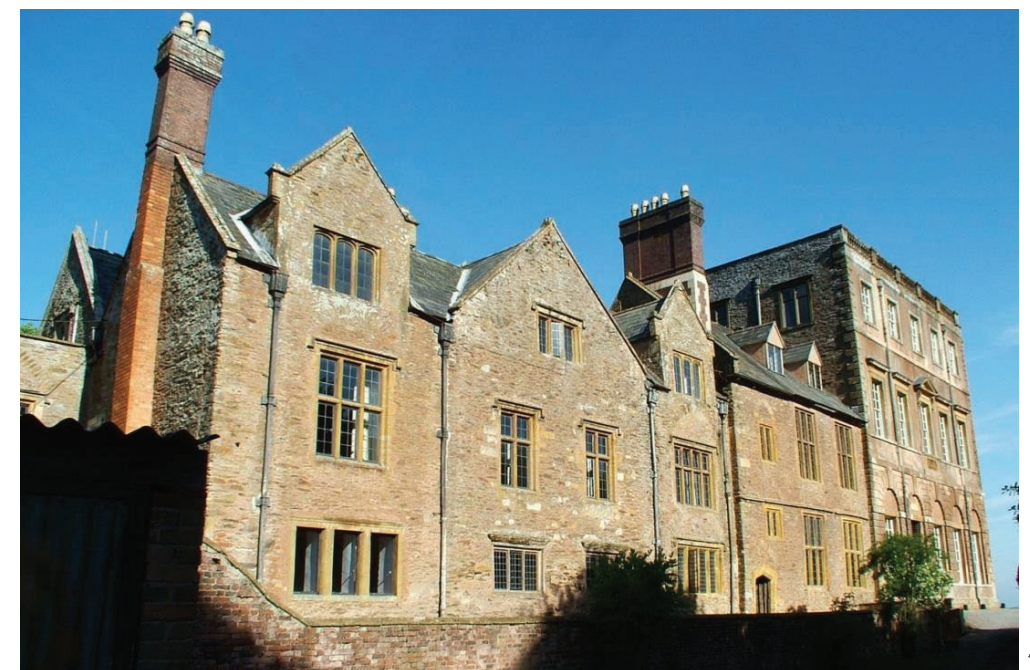
Fig. 2.27. c. 2006, east façade with new mullions of c. 1926.
