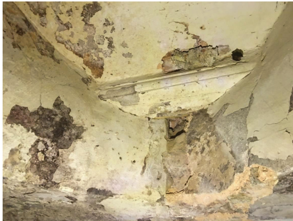
Fig. 5.18. An ovolo-moulded piece of masonry, reused in the construction, or blocking-up, of the ceiling opening to in the south-west of the southern chamber. The blocked opening would have led to the courtyard before an extension of 1754 brought that area within the house.
