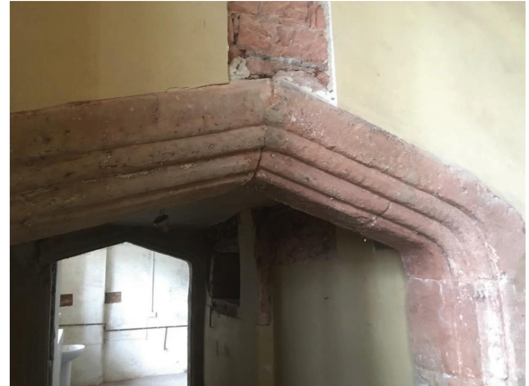
Fig. 2.21. Two similar four-centred arch door surrounds of red sandstone leading from the inner porch to the Hall and the Kitchen. Both doors are decorated only to their north, Hall-facing, sides with ironmongery to the undecorated south sides.
