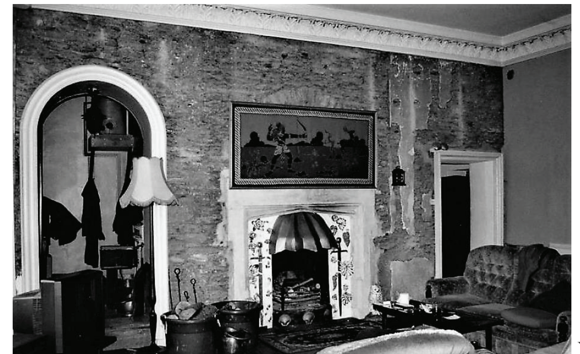
Fig. 2.11. Halswell, the Solar above the Hall in c. 1980, with a late sixteenth-century fire surround (with later additions) and relieving arch above. The wall is punctuated with fixing holes for panelling.
