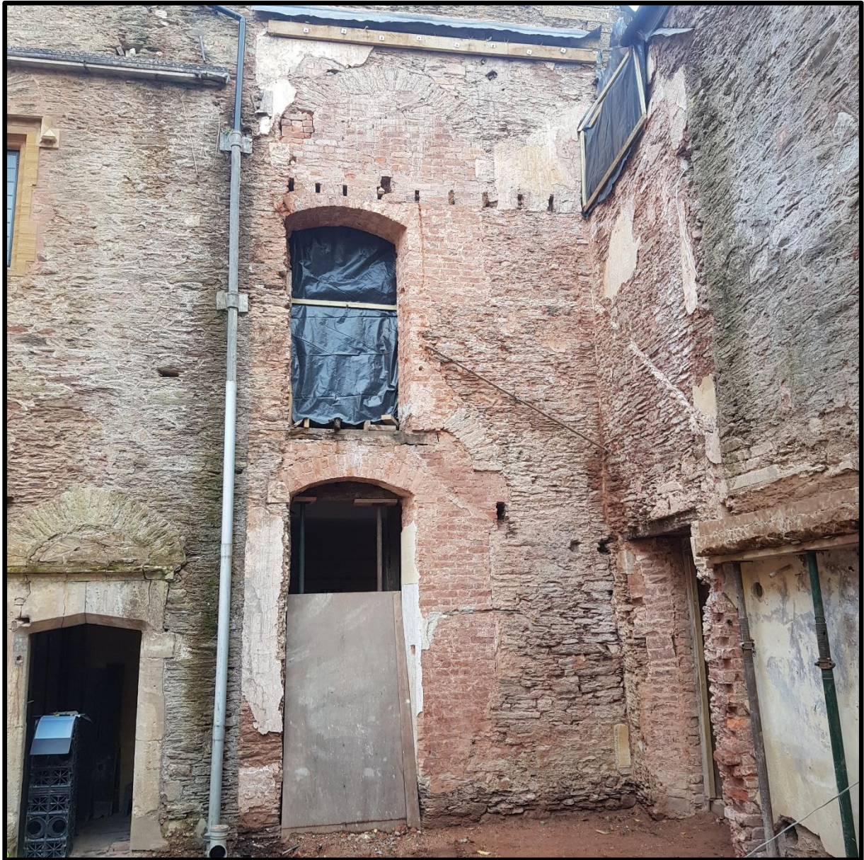
General view of the west elevation of the east range showing the projecting partial foundation of a possible earlier stair structure, the position of two earlier window openings, the position of the two later windows, and the late 18 th century staircase arrangement. Looking east.
