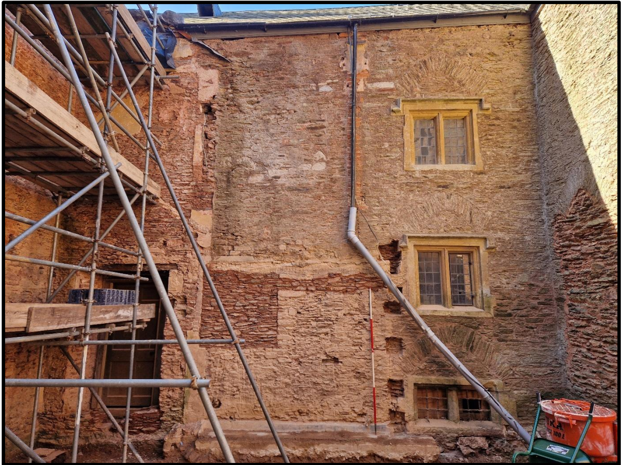
General view of the north elevation of the south range showing the partial position of the earlier window on the ground floor. 2m scale. Looking south.
