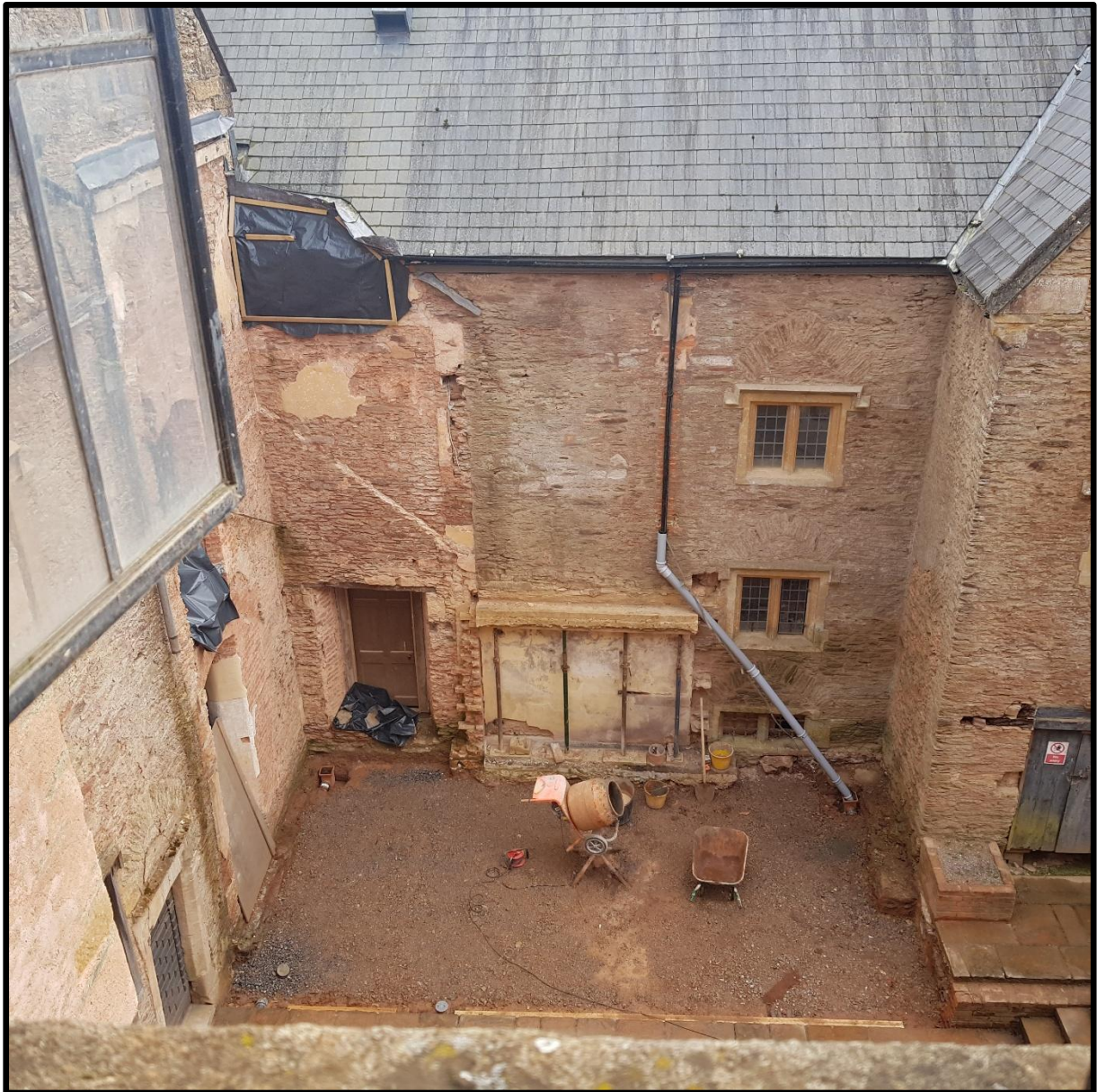
General view of the north elevation showing the position of two earlier windows, the remains of a possible pentice, the position of an earlier ground-floor window and later inserted doorway. Looking south.
