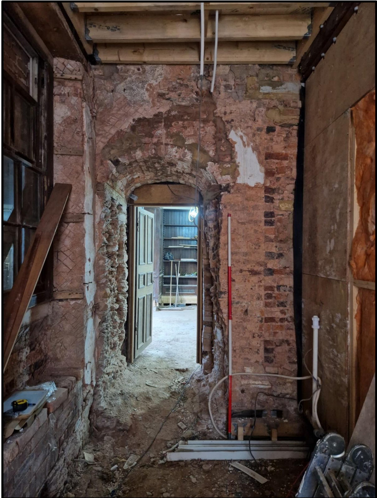
General view of the opening between G49 and G39 showing the earlier projecting brickwork to the right and the later arched opening (centre). 2m scale. Looking north.
