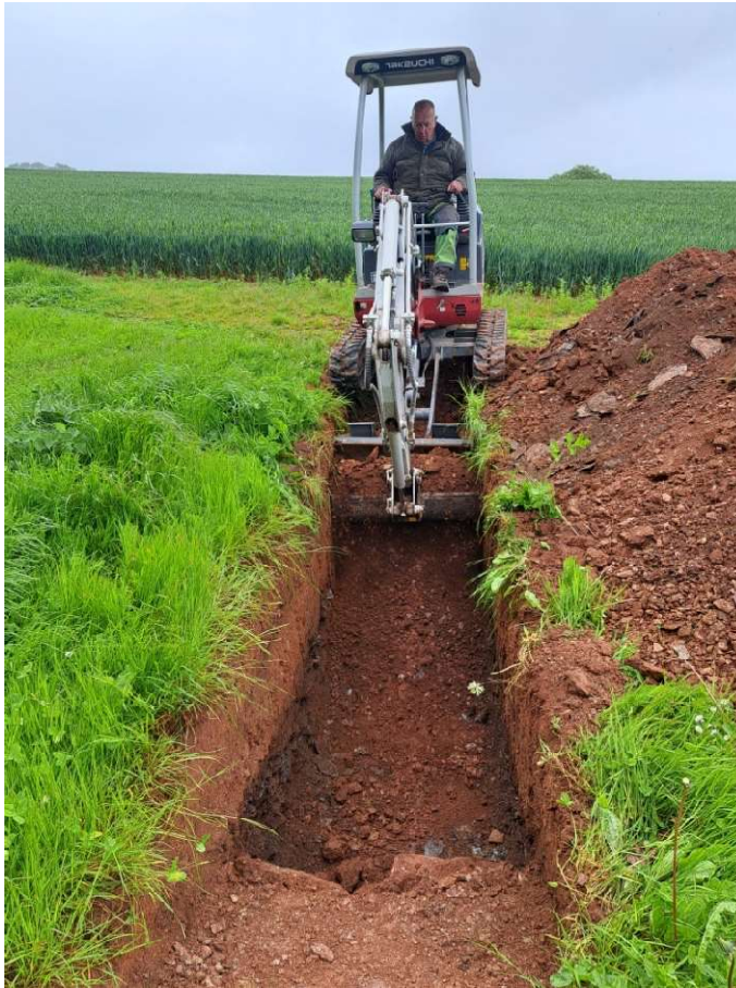
Pl. 1: Commencement of excavation in Trench 1 to the west of the site (view from E)
