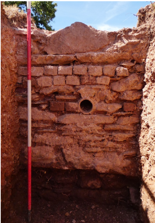
Pl. 10: East facing elevation of retaining wall (405)/(406) in Trench 4 (view from E; scale=1.50m)
