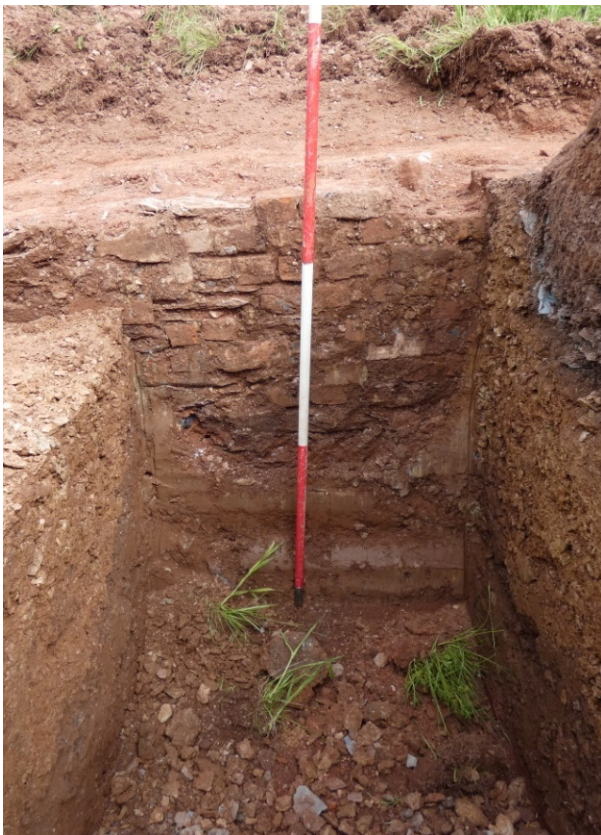
Fig. 5: Detail exposed elevation of retaining wall (106) & repair (112); Area 1 central (view from W; scale=1.50m)
